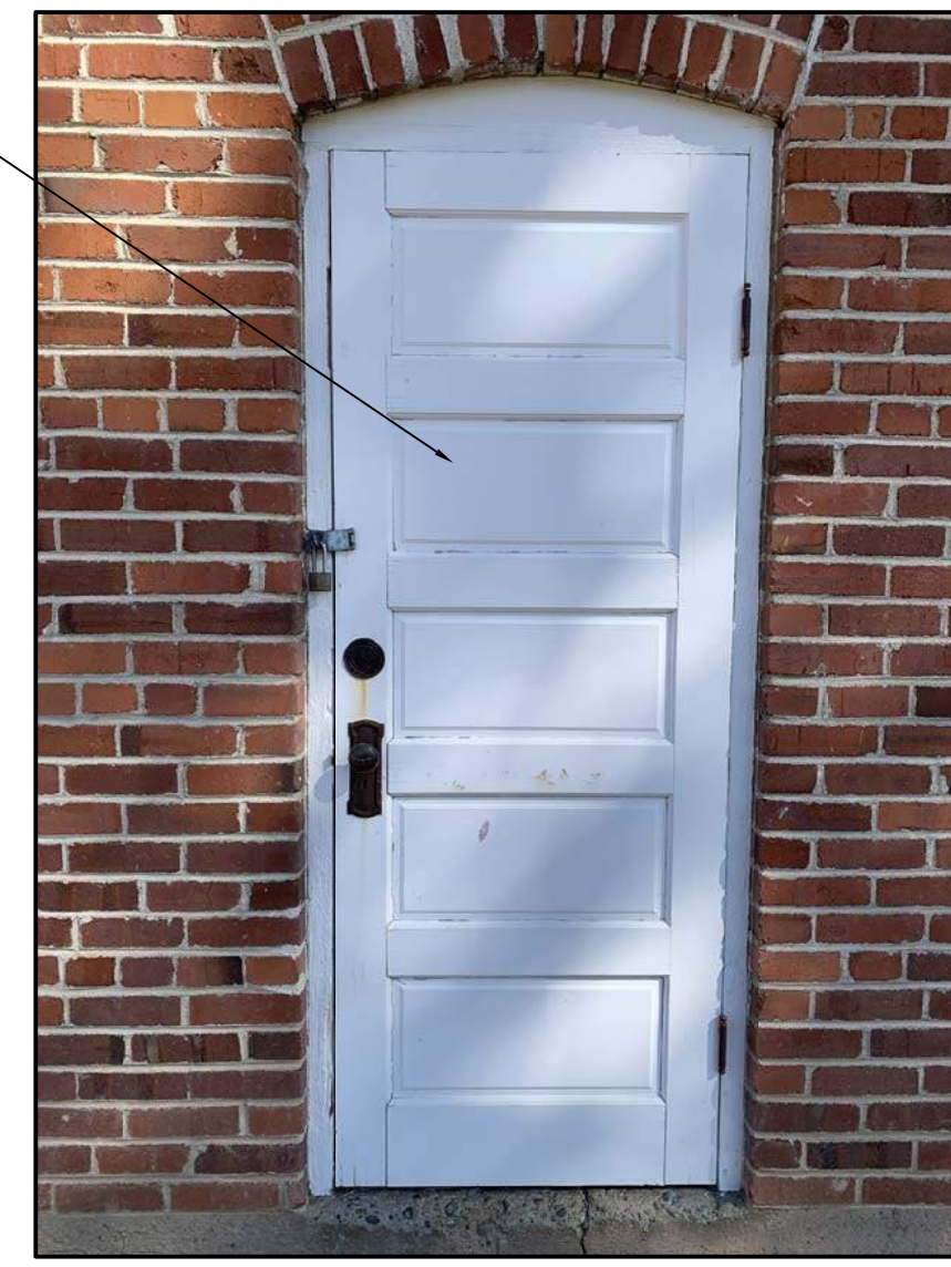
A2 Photo of Existing Condition N.T.S.
