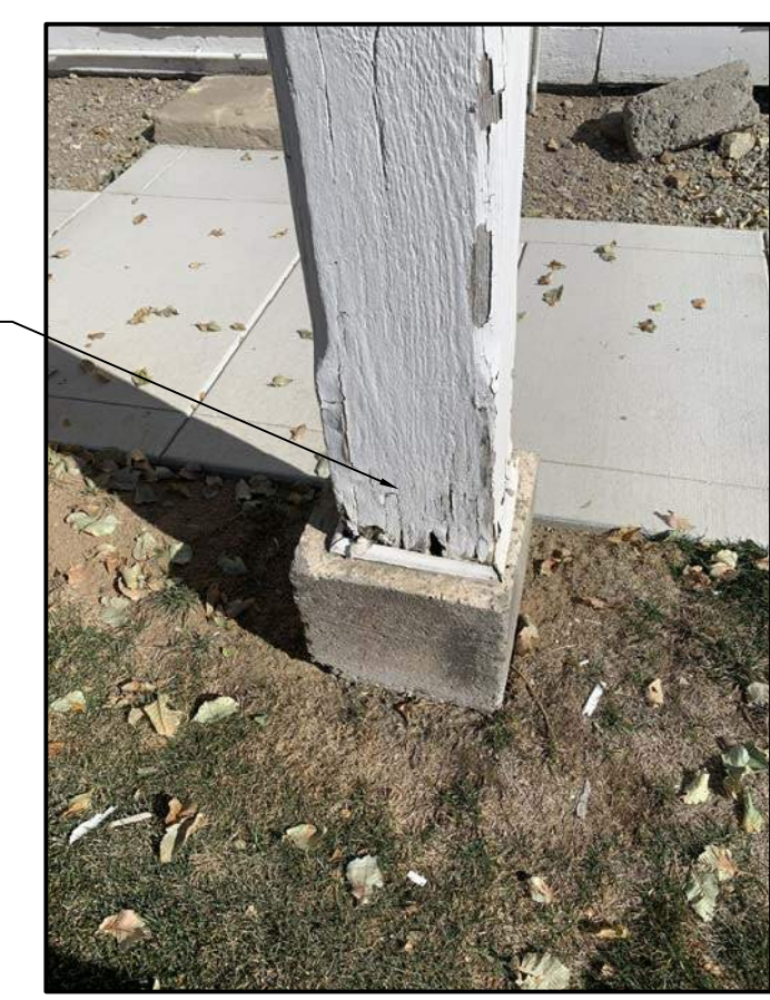
B2 Photo of Existing Condition N.T.S.
