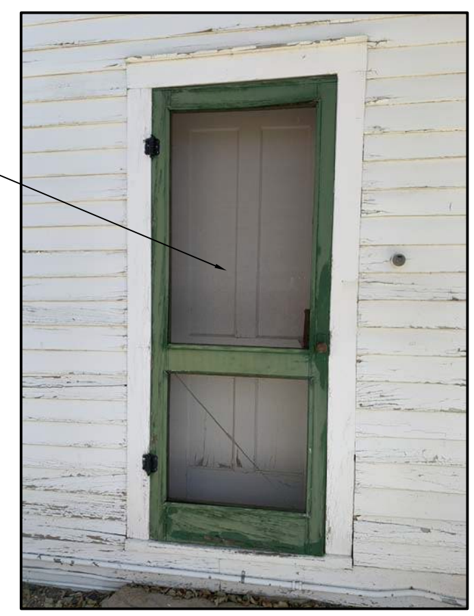
B3 Photo of Existing Condition N.T.S.
