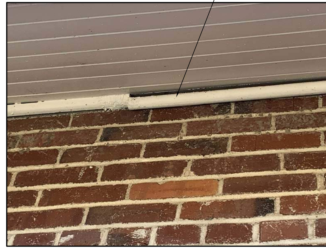
A3 Photo of Existing Condition N.T.S.
