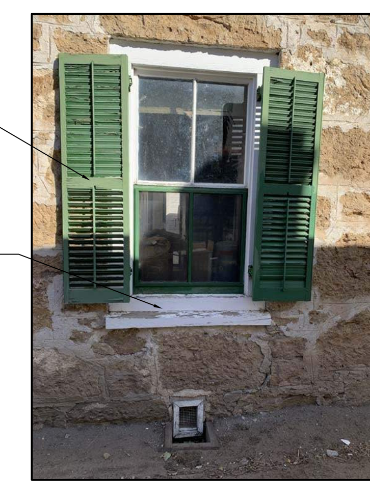
A2 Photo of Existing Condition N.T.S.
