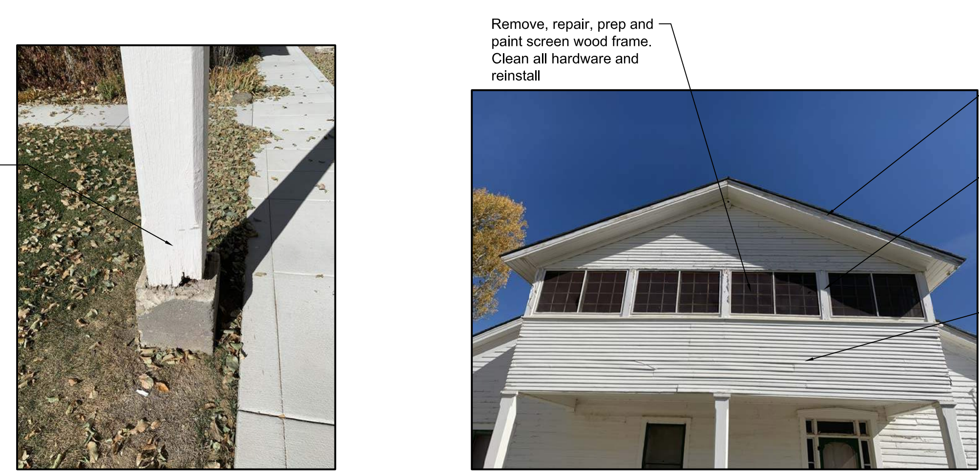
A4 Photo of Existing Condition N.T.S.
