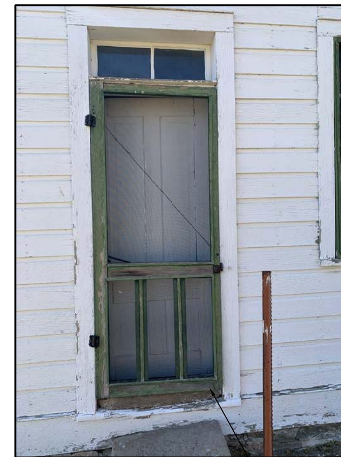
A2 Photo of Existing Condition N.T.S.
