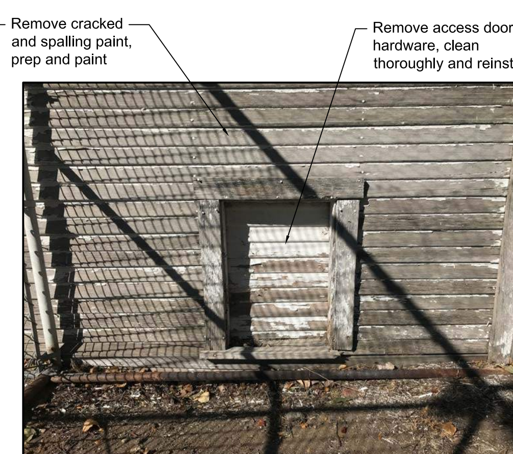
B3 Photo of Existing Condition N.T.S.
