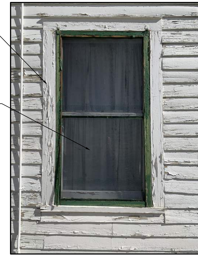
B1 Photo of Existing Condition N.T.S.
