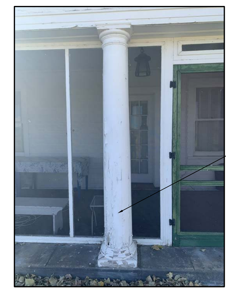
B4 Photo of Existing Condition N.T.S.
