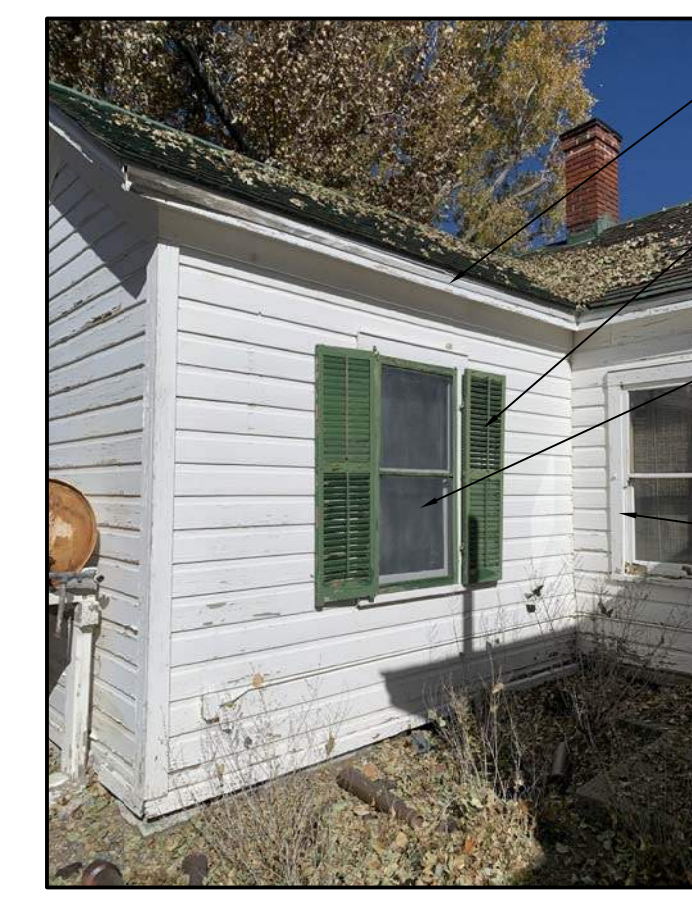
B5 Photo of Existing Condition N.T.S.
