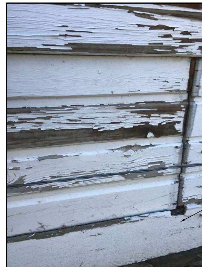
A3 Photo of Existing Condition N.T.S.
