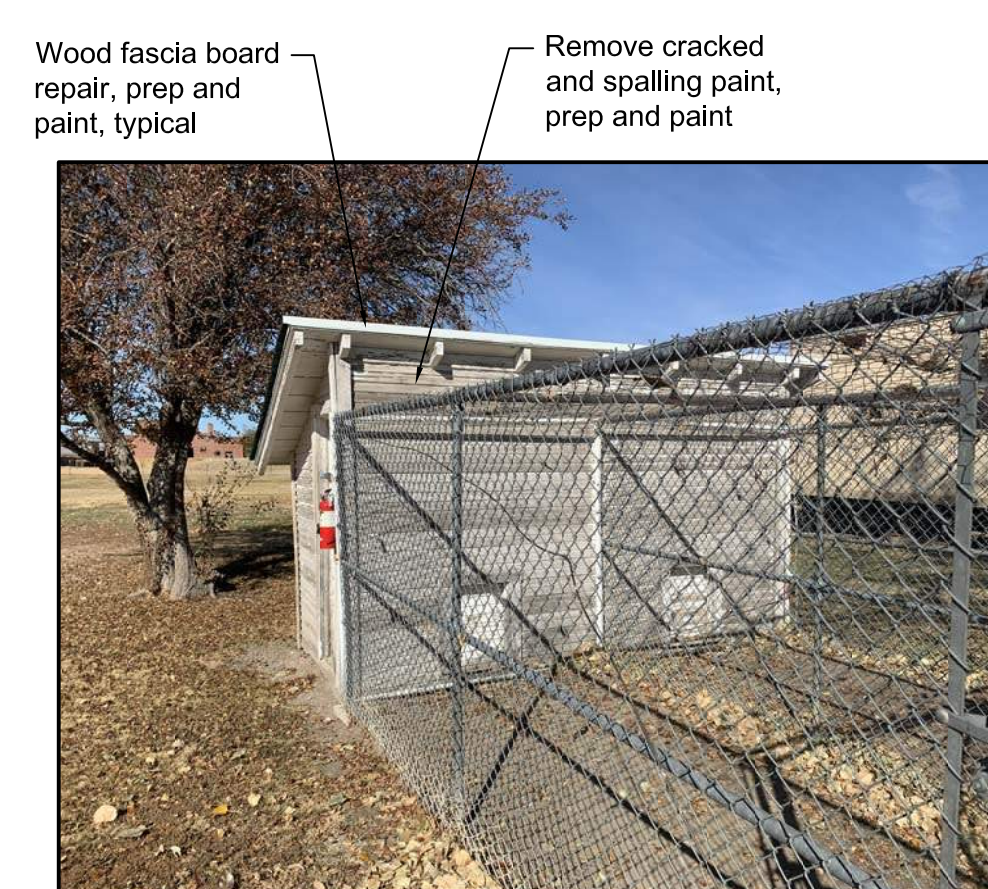
B2 Photo of Existing Condition N.T.S.
