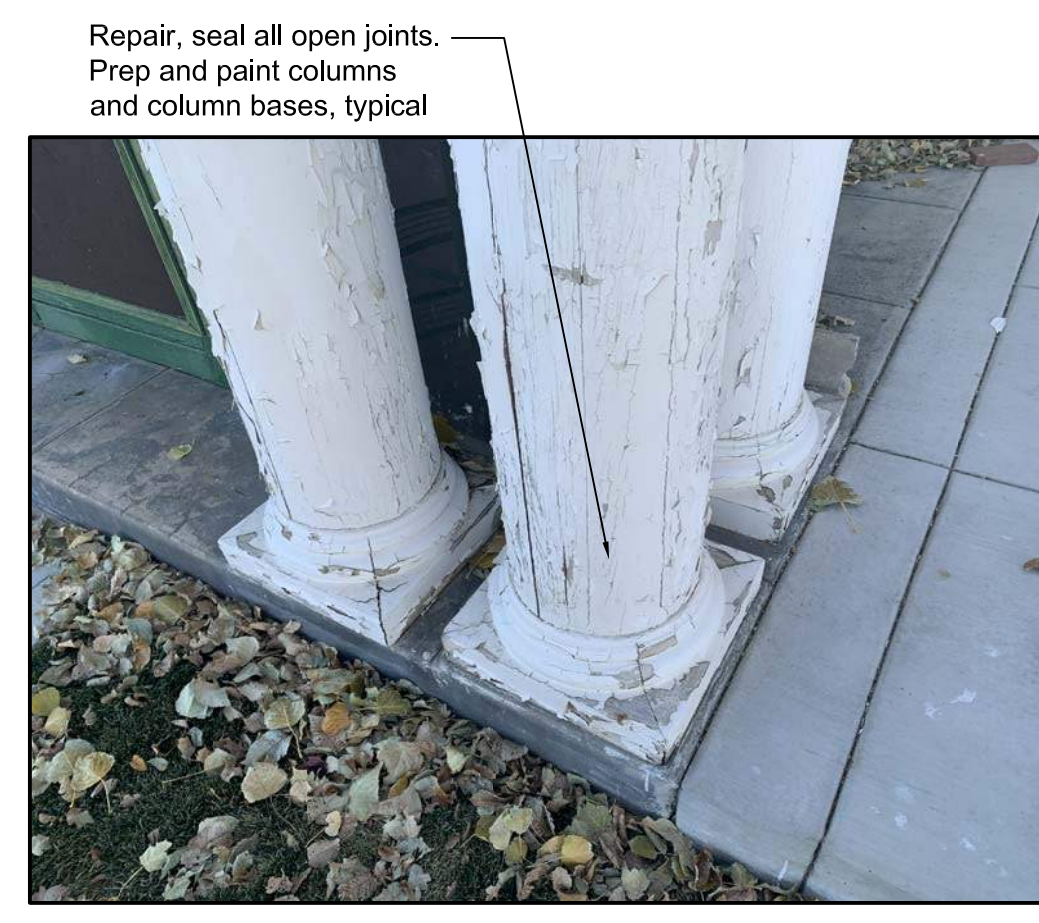
C1 Photo of Existing Condition N.T.S.
