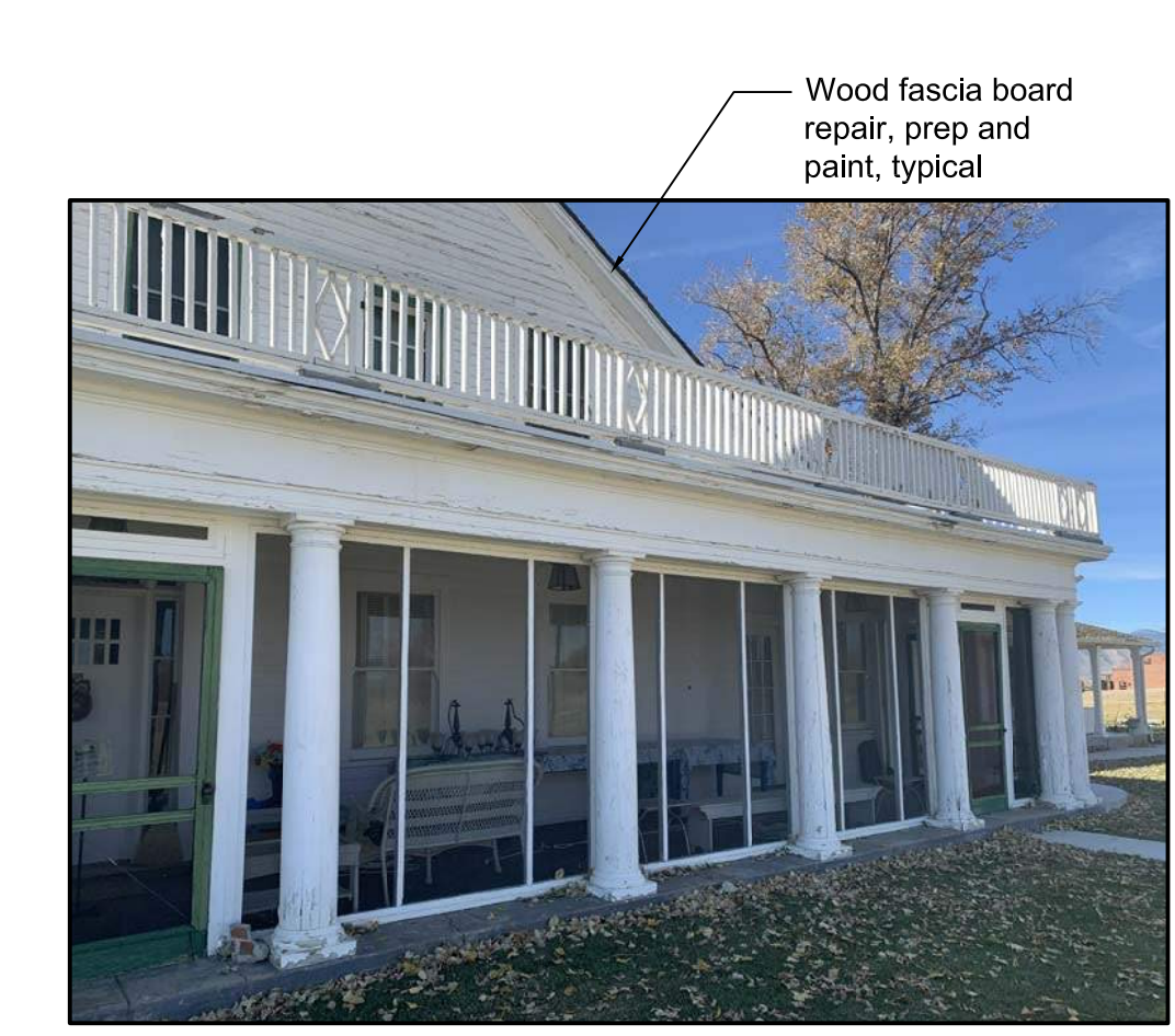
C2 Photo of Existing Condition N.T.S.
