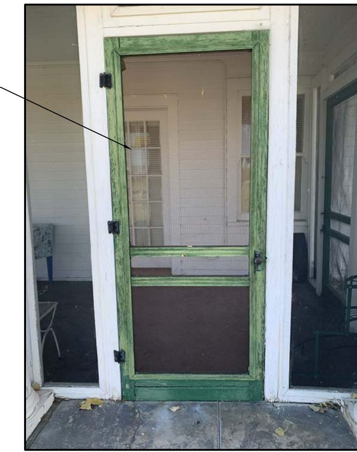
B3 Photo of Existing Condition N.T.S.
