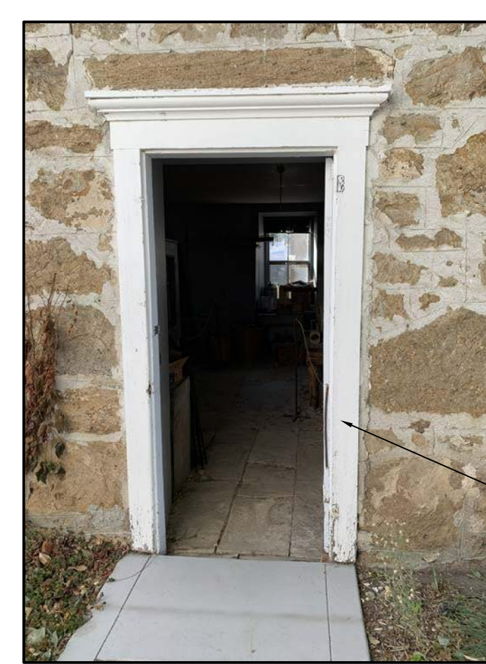
A3 Photo of Existing Condition N.T.S.
