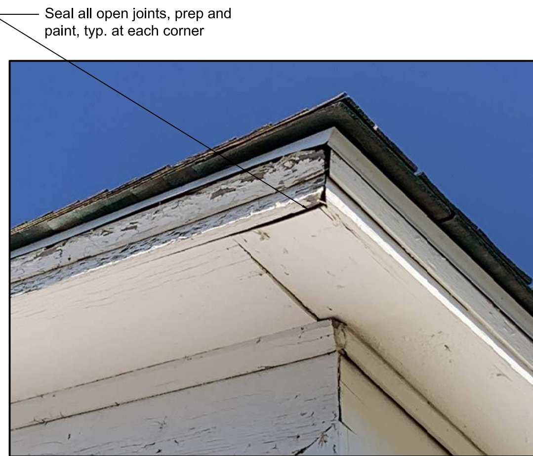
A4 Photo of Existing Condition N.T.S.
