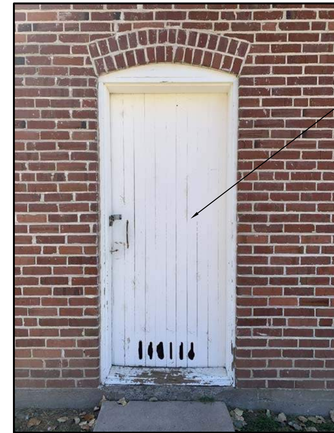
B5 Photo of Existing Condition N.T.S.
