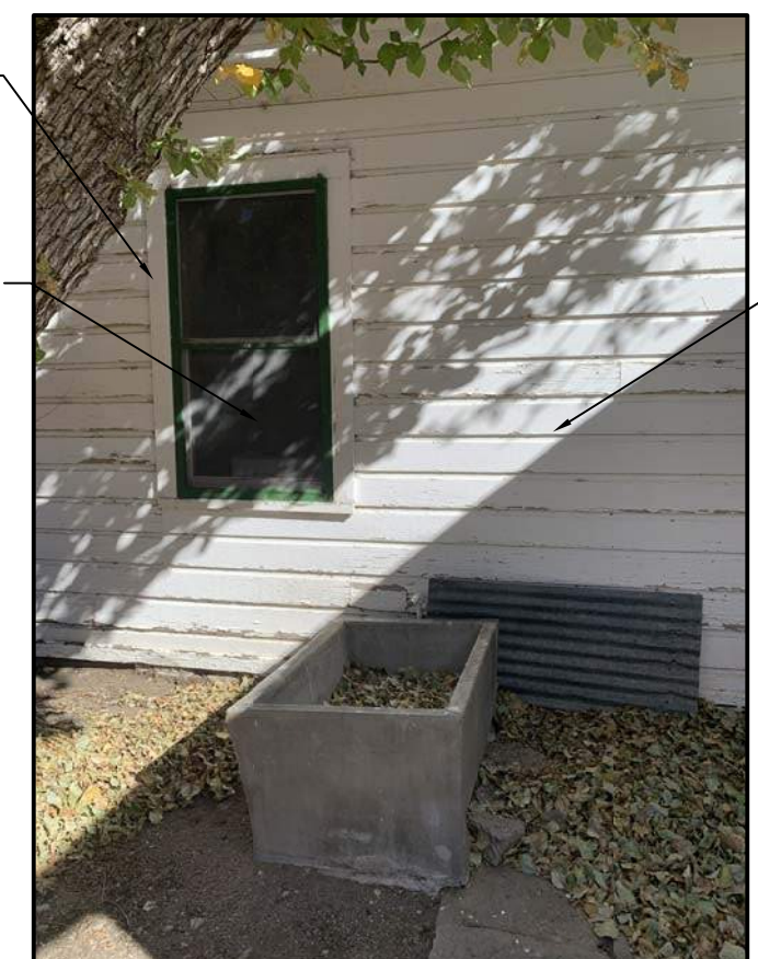
C3 Photo of Existing Condition N.T.S.
