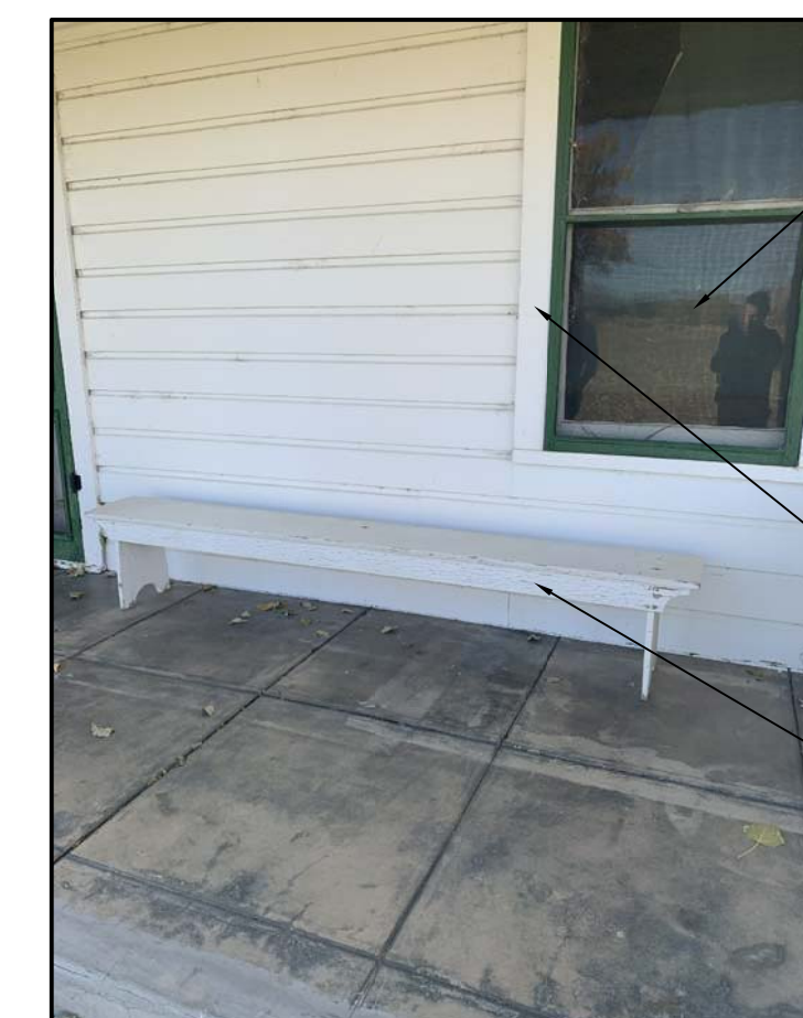
A3 Photo of Existing Condition N.T.S.
