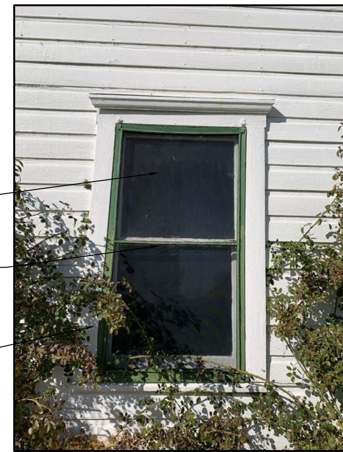
A4 Photo of Existing Condition N.T.S.
