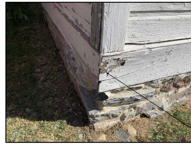
B5 Photo of Existing Condition N.T.S.
