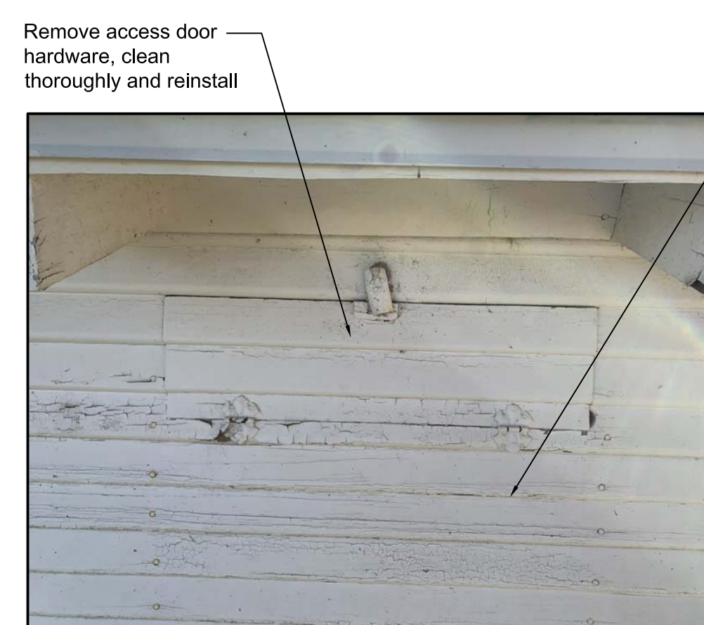
B4 Photo of Existing Condition N.T.S.
