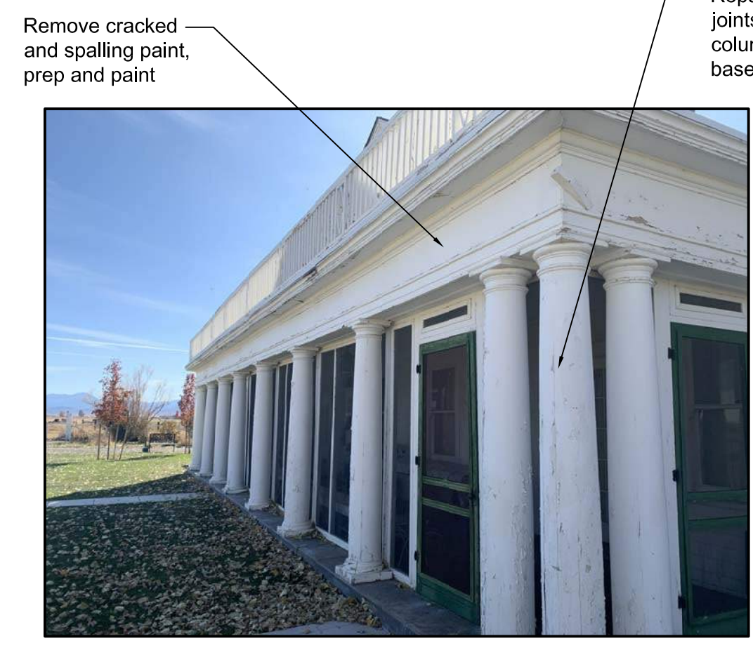
B2 Photo of Existing Condition N.T.S.
